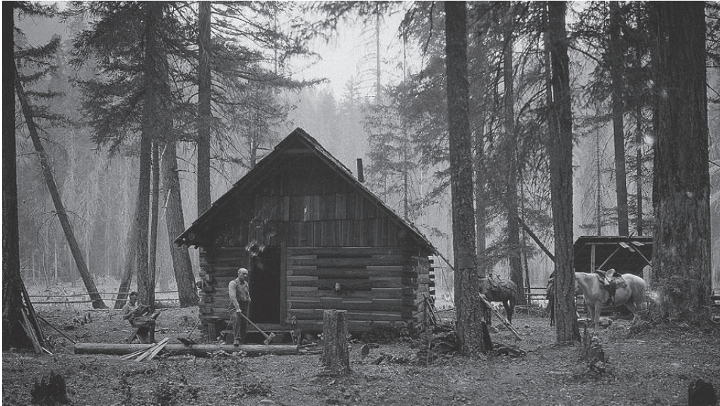
Cabin being built in Region 6, Umpqua National Forest 1922
