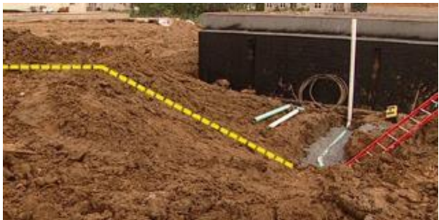
Trenching and Excavation Toolkit
