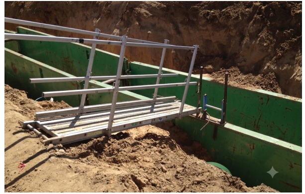
Adequate access and egress also includes access to the edge of the trench where the protective system is removed from the edge.
