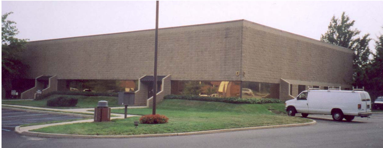
Figure 2. Moisture investigation of a single-story flood. A water heater broke, flooding the floor in this office condominium over a weekend. Water seeped up into walls through capillary action, for more than 48 hours.
