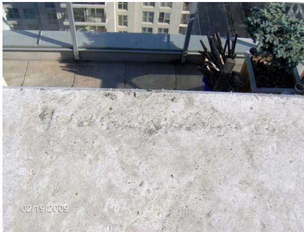
PHOTOGRAPH 5: The ellipse denotes an area where the silicone paint has delaminated from the concrete slab.
