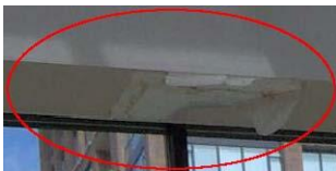
PHOTOGRAPH 12: Exterior view of a raised leg skylight with overlapped drainage gutters.
