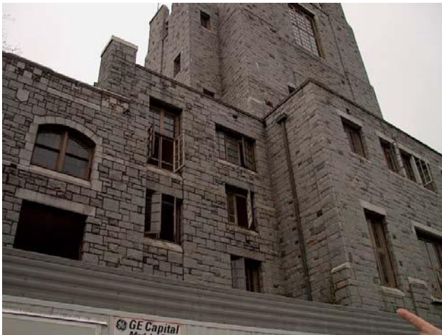
Photograph 1: Closed-cell spray applied polyurethane foam was utilized on the interior side of the cast-in place concrete wall as insulation during the retrofit of this building in 2005.
