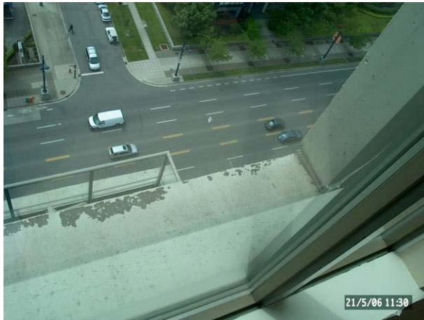
PHOTOGRAPH 2: View of the outward projection of a floor slab from the interior of the building. Note the spalling paint on the surface of the slab.
