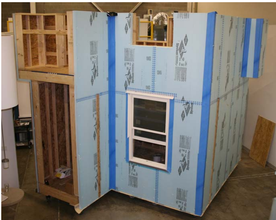
Figure 2. Wall mock-up constructed and sheathed. The 2x6 wall system is in the foreground.
