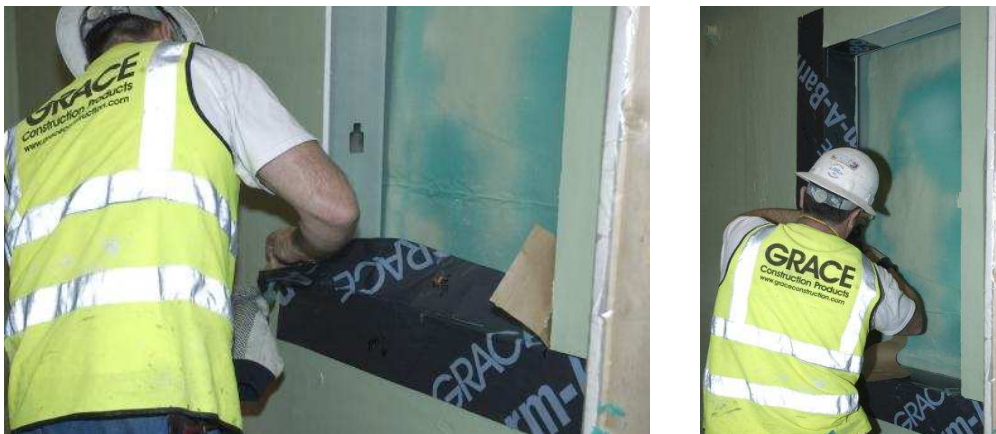
Figure 8: Flashing windows with a fully adhered membrane.
