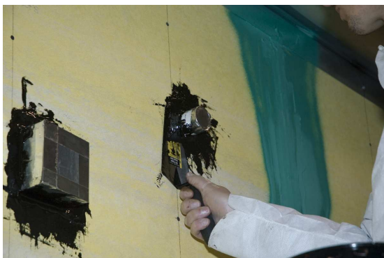
Figure 6: Application of sealant at PVC pipe and HVAC duct penetrations.
