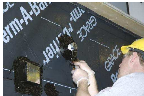
Figure 6: Application of sealant at PVC pipe and HVAC duct penetrations.
