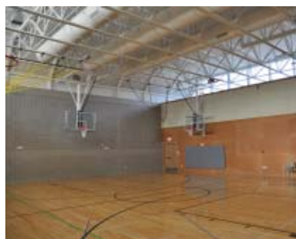
Figure 23: Gym looking through north clerestory and light shelf
