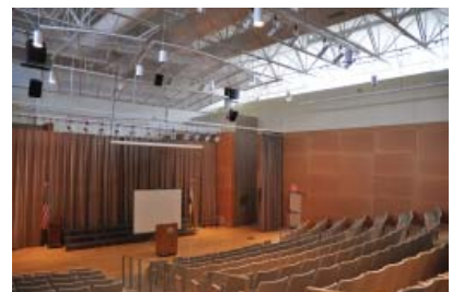
Figure 25: Auditorium looking at southeast clerestory and light shelf
