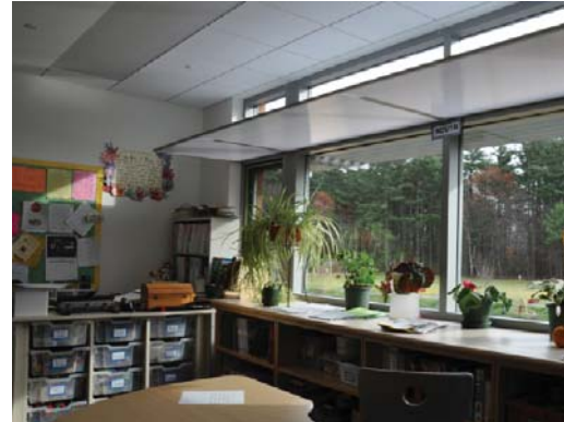
Figure 15: Interior light shelf at classroom
