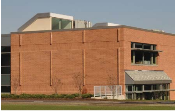
Figure 17: Exterior view of south facing classroom wing looking northeast showing clerestory roof monitor at back of upper level
