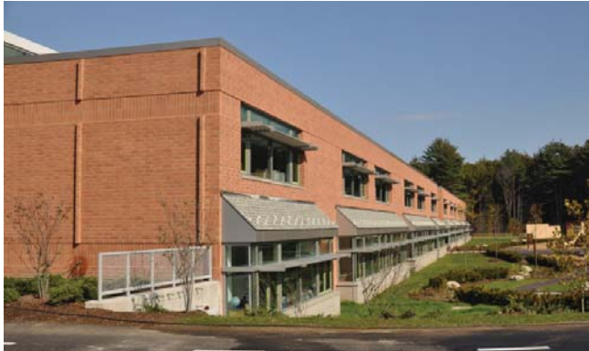
Figure 14: Sunshades at South Facade of classroom wing looking east
