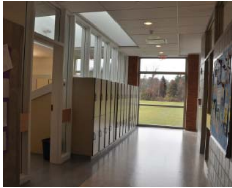
Figure 19: Upper level classroom corridor looking at slot in ceiling for shared clerestory daylight
