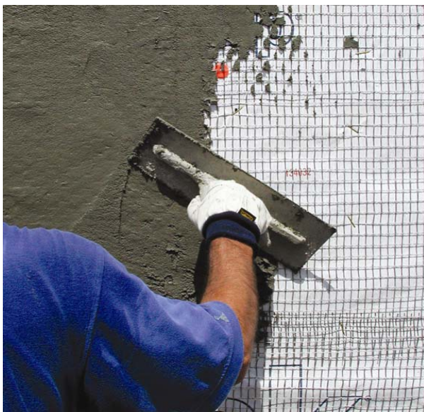
Figure 2 PermaLath Glass Fiber Lath
