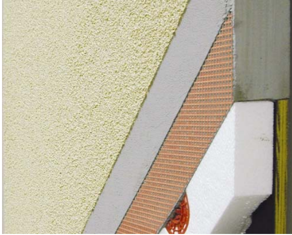
Figure 1 EIFS with woven fiberglass mesh
