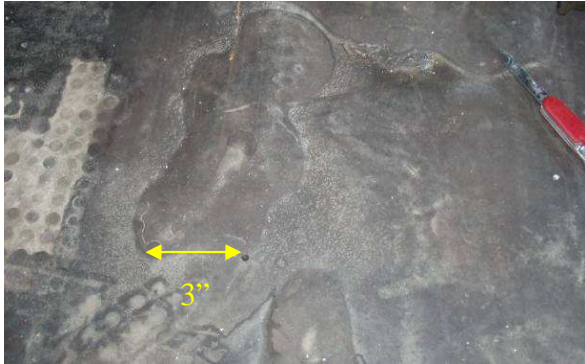
Figure 1 & Figure 2: Typical Blistered Roof Membranes. Blister size ranging from penny sized blisters to areas several square feet, membrane 5-10 years old.
