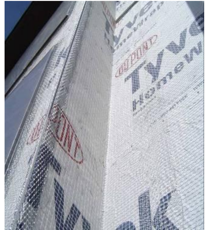
Installed Plaster Base
