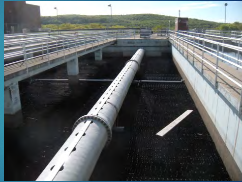
Settling Basin 35 MGD Flow Rate/Basin
