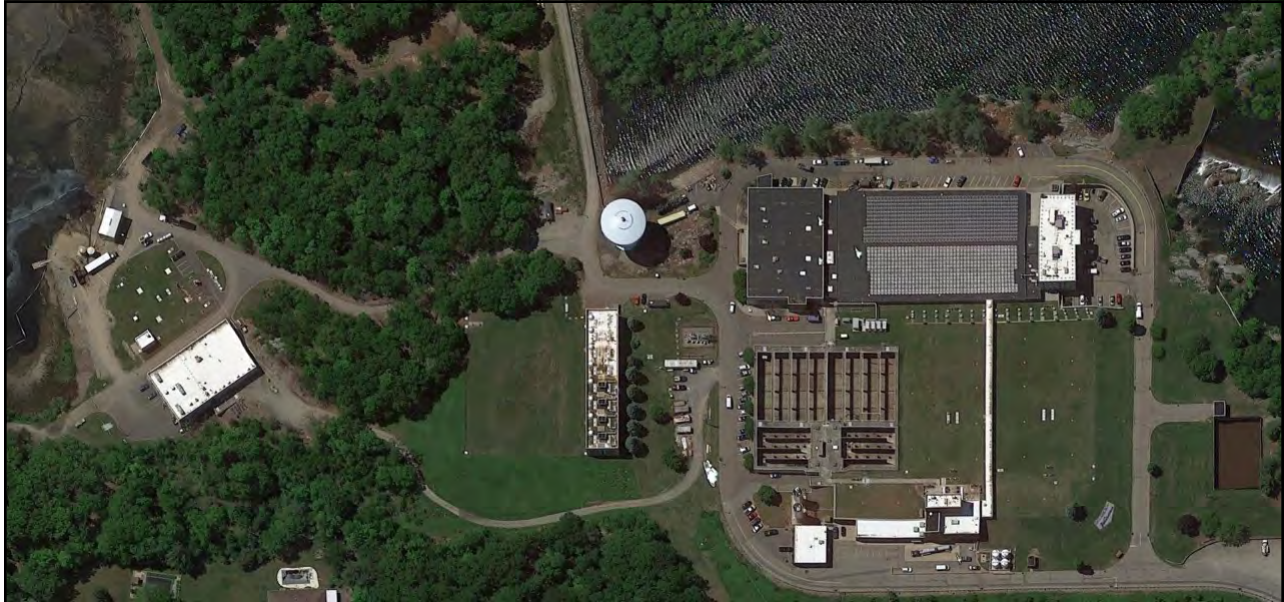
North Jersey District Water Supply Commission (NJDWSC) Upgrades Two of Their Clarification Basins
