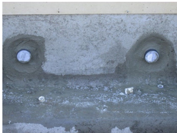
Plumbing with fittings installed and pre-sealed.
