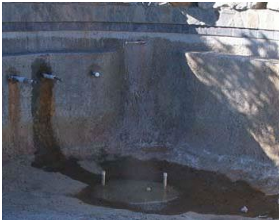
Water from behind the structure prior to application of the interior finish coating.
