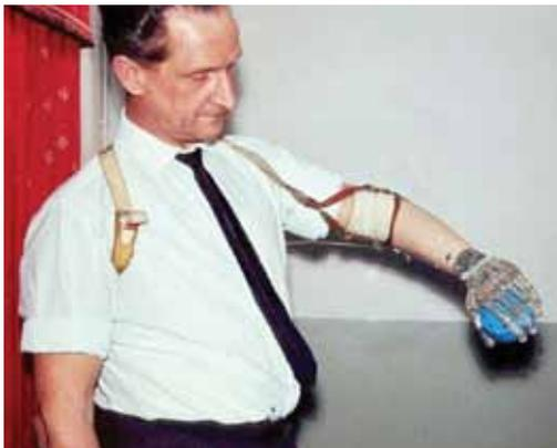
**Figure 1:** Patient Bob Daish uses a cable-operated, multi-articulated hand in the 1960s.
