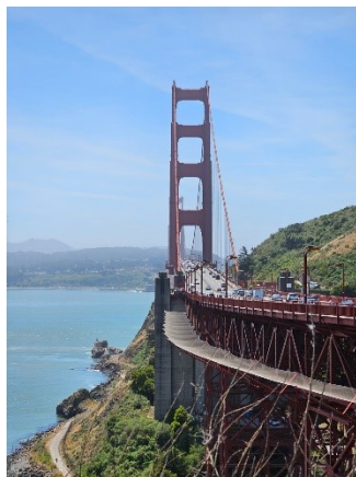
Golden Gate Bridge
