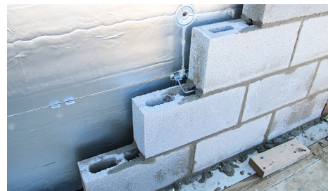
Polyiso wall insulation on a commercial building.
