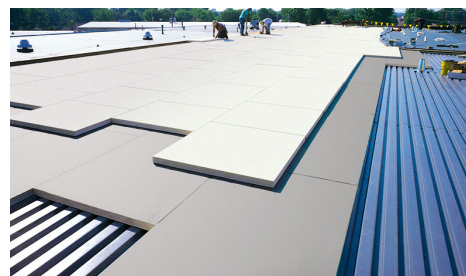
Polyiso roof insulation on a commercial building.
