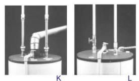
heater. CPVC is approved by all the model codes for use as relief valve drain line piping. Use a metal-to-CPVC transition fitting to connect to the relief valve and continue the pipe full size to the outlet. For horizontal runs, slope the pipe toward the outlet and support it at three-foot centers or closer. The pipe must discharge to the atmosphere at an approved location.
