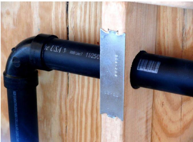
*ABS DWV system with solvent welded joints*
