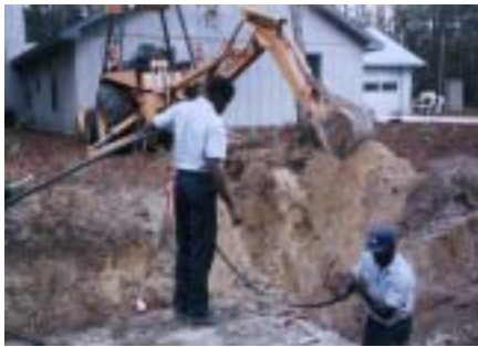
Installation of PE pipe in trench.
