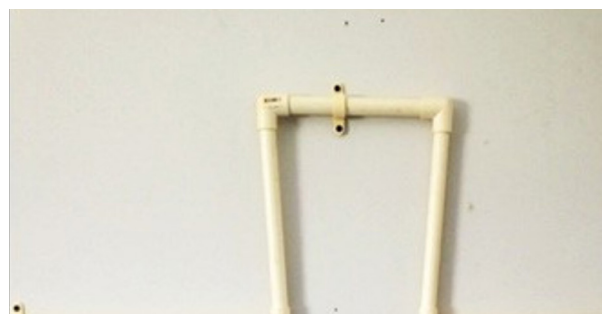
Image 9. Proper Offset Loop Design Allows Movement
