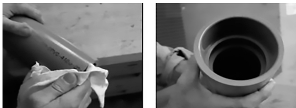
Images 11 and 12. Fitting Preparation
