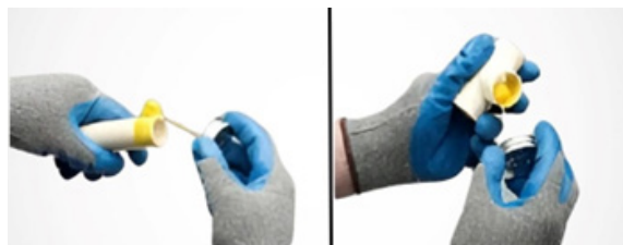
Images 6 and 7. Cement Application
