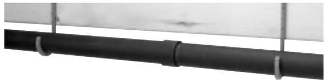
ABS pipe should be supported similarly to other piping systems using pipe hangers. Avoid hangers that may cut or compress pipe and tight clamps or straps which prevent pipe from moving or expanding.
