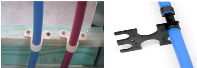
*PEX tubing with check gauge in hot and cold water distribution.*
