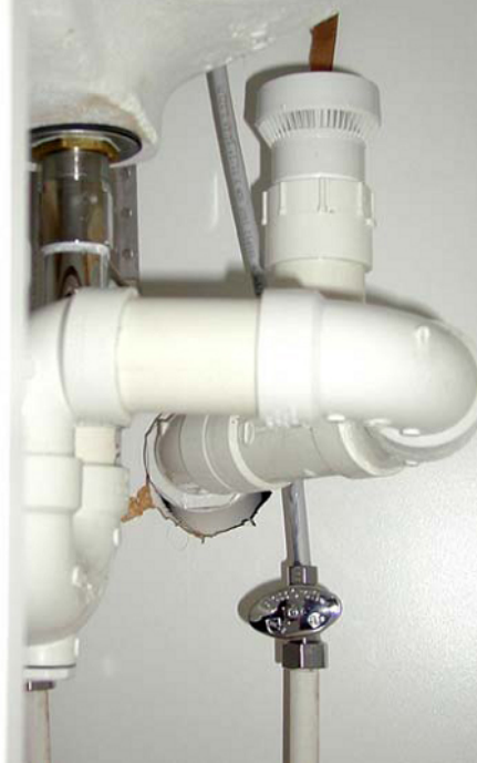
Figure 75. An Installed Air Admittance Valve
