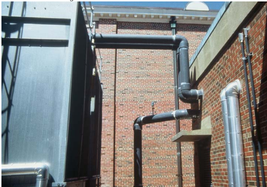
Figure 86. Outdoor Condenser Return Lines
