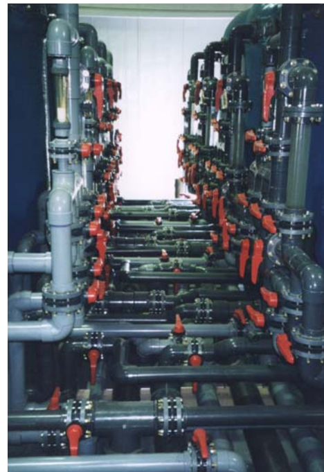
Figure 20. PVC Pipes Transporting Chemicals
