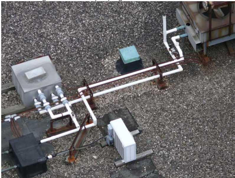
Figure 94. Rooftop Piping with Condensate Drain
