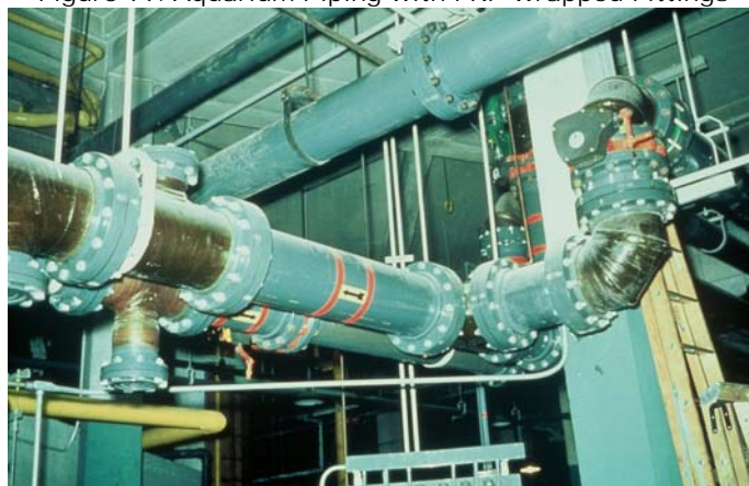
Figure 99. Aquarium Piping with FRP Wrapped Fittings
