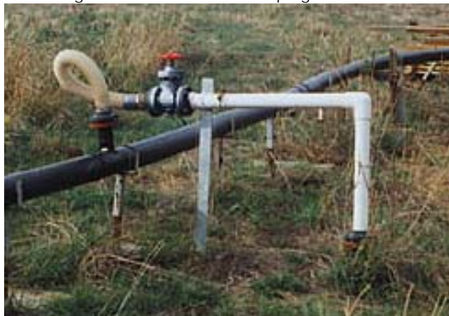
Figure 103. Odor Control Piping at Landfill
