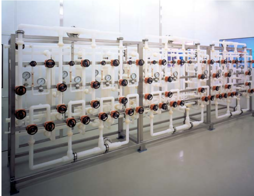
Figure 134. High Purity Water Piping System
