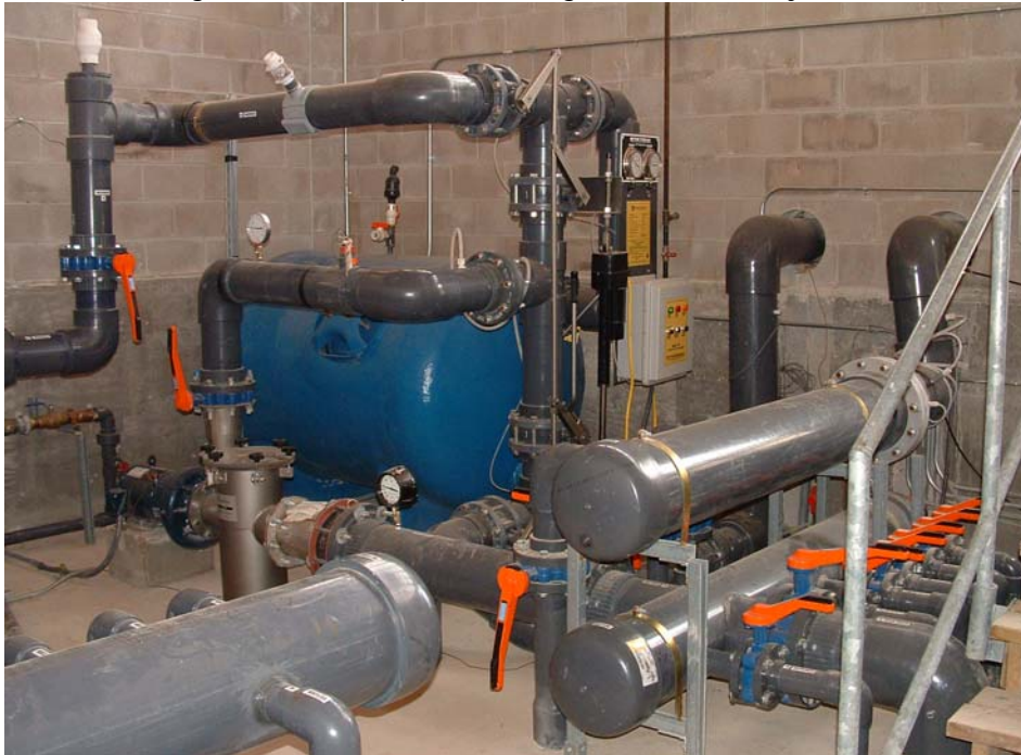
Figure 111. Municipal Swimming Pool Filtration System
