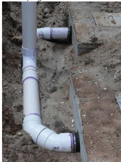
Figure 92. Piping for Restaurant Grease Traps
