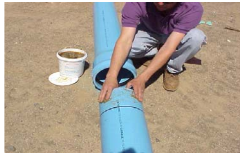
Figure 63. Gasketed Joint Assembly
