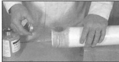
Figure 59. Solvent Cementing
