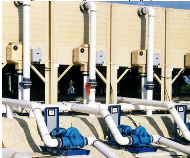
Figure 88. Cooling Tower Pumping System
