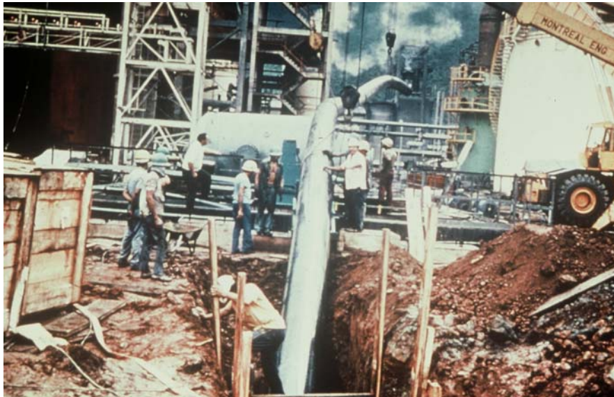
Figure 129. Power Plant Intake Piping Line
