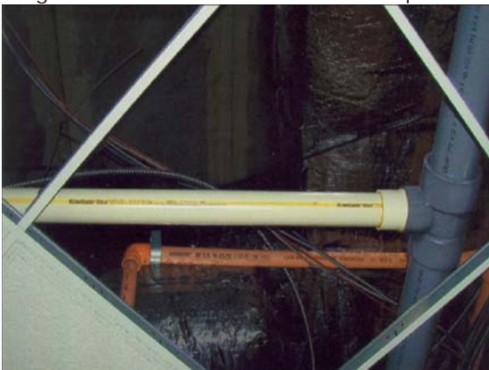
Figure 126. Hot/Cold Water and Fire Sprinkler
