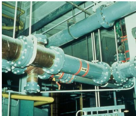
Figure 18. Aquarium Piping with FRP Wrapped Fittings in Use for Over Four Decades
