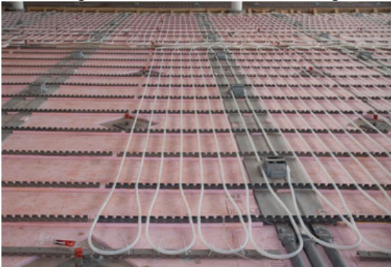
Figure 130. Radiant Floor Heating
