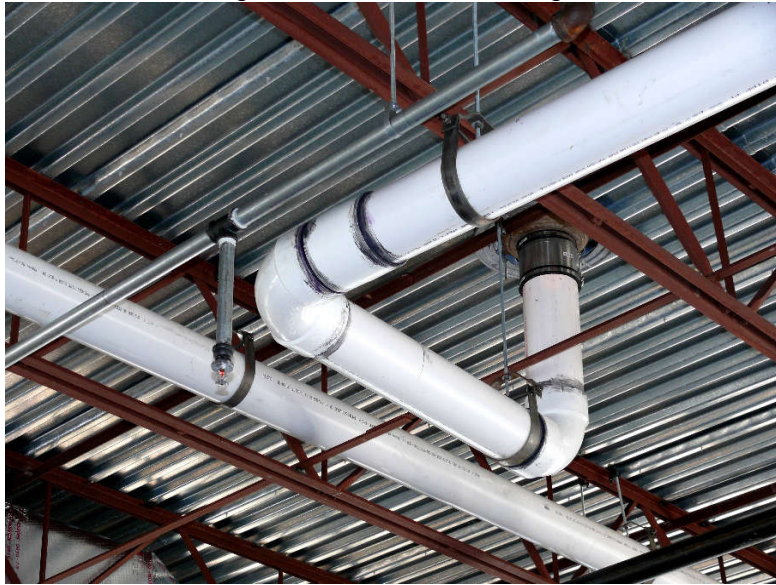
Figure 93. Storm/Roof Drainage
