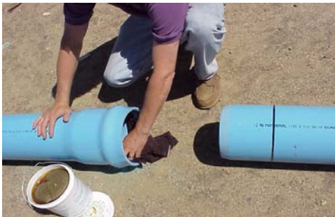
Figure 63. Gasketed Joint Assembly
