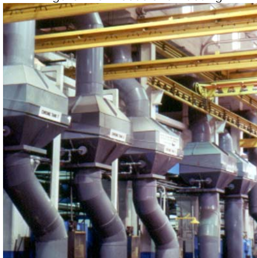
Figure 115. Hoods and Ducting
