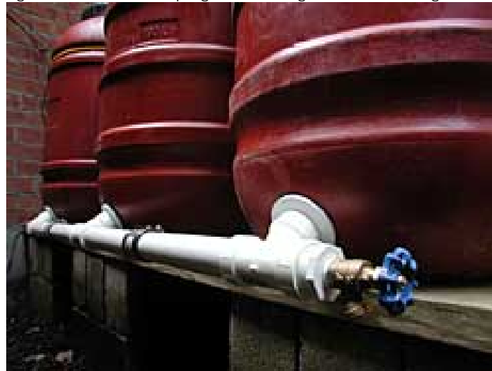
Figure 96. Manifold Piping Connecting Rain Harvesting Barrels
