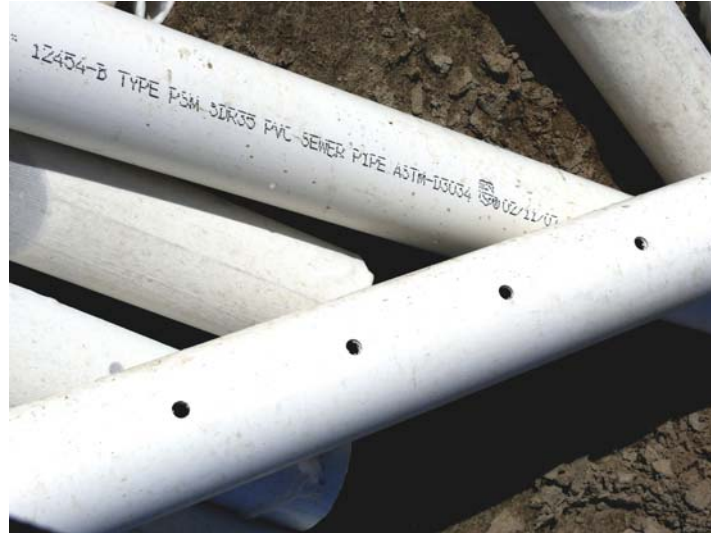
Figure 95. Subsoil Drainage
