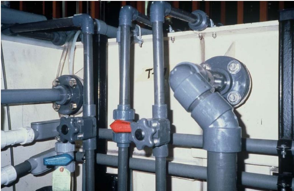
Figure 112. Bleach Process Piping
