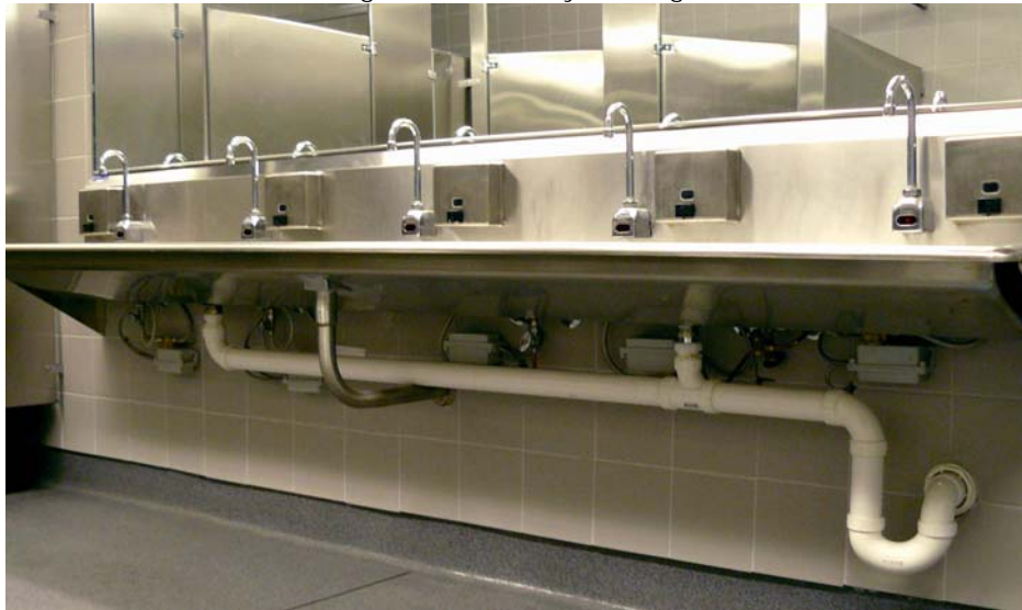
Figure 90. Sanitary Drainage
