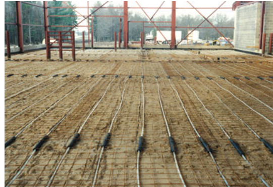
Figure 131. Permafrost Protection
