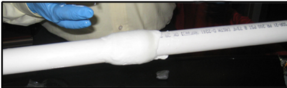
The finished product repair requires curing before testing.
