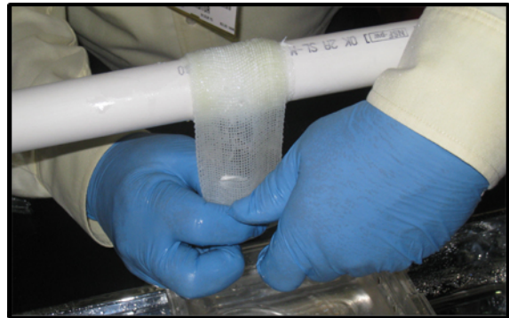
Final wrapping of repair Notice the use of latex gloves during installation.
