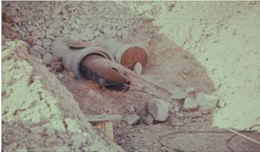
Figure 25. Pipe Lining
