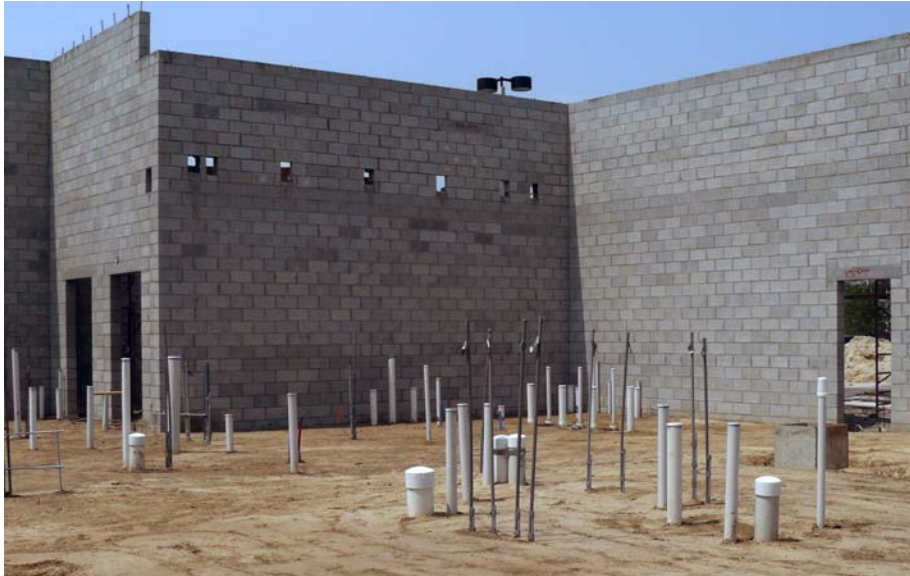
Figure 89. Drainage, Waste, and Vent Piping at a Commercial Job Site
