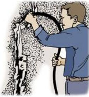
**FIG. 7** - Moistening the area to be repaired prevents the newly applied patch from drying out.
