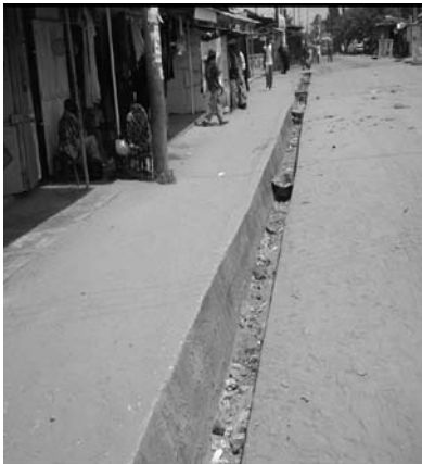
Figure 1: Murrum road with storm water drain (January 2005) Source: Authors
