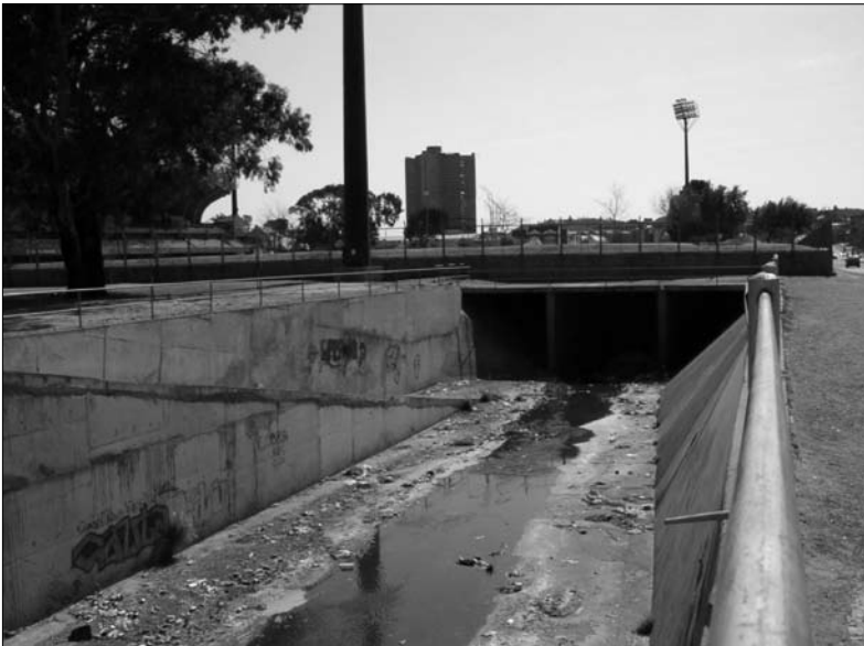
Figure 3: Storm water channels which increase the speed of the storm water Source: Steenkamp, 2008: own picture
