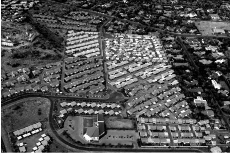
Figure 2: Homogeneous residential developments Source: Steyn & Schoeman, 2006: CD- ROM
