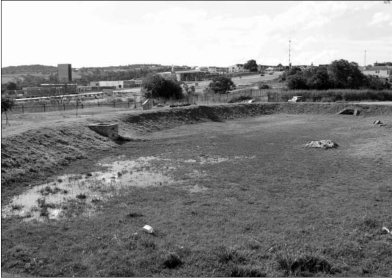
Figure 1: Typical open-air storm water attenuation pond in the Johannesburg area. Source: Aldous, 2007: own picture
