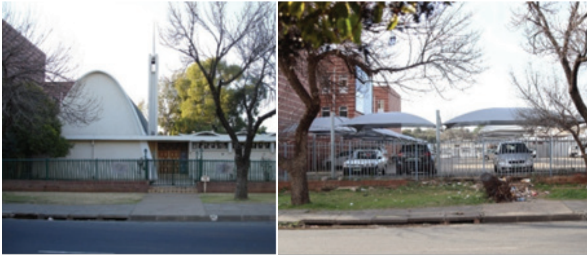
Roberts and Cassells ca 1956. The southern side of Chapel of the CLDS viewed from Nelson Mandela Drive Source: Du Preez, 2005
