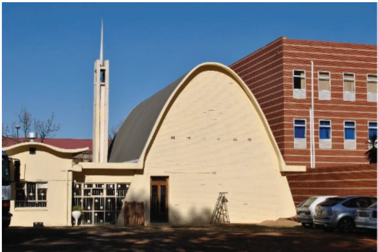
Figure 2 Photograph of the Northern Elevation of the Chapel 2013
