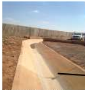
Concrete lined trench
