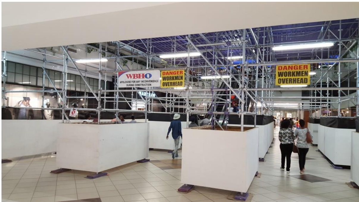
Photo: ‘Better Practice’ Construction H&S, Greenacres Shopping Centre, Port Elizabeth (Smallwood, May 2016)
