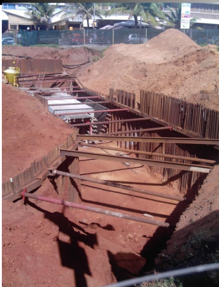
Culvert construction within a trenched sheeted excavation, uMhlanga (Smallwood, 2007)
