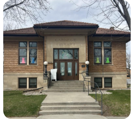
Armour Carnegie Public Library
