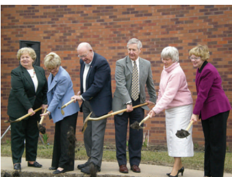
Marcie Moran, Carol Twedt, Bob Jamison, Mayor Dave Munson, De Knudson, & Library Director Sally Felix break ground on the Siouxland renovation & expansion.
