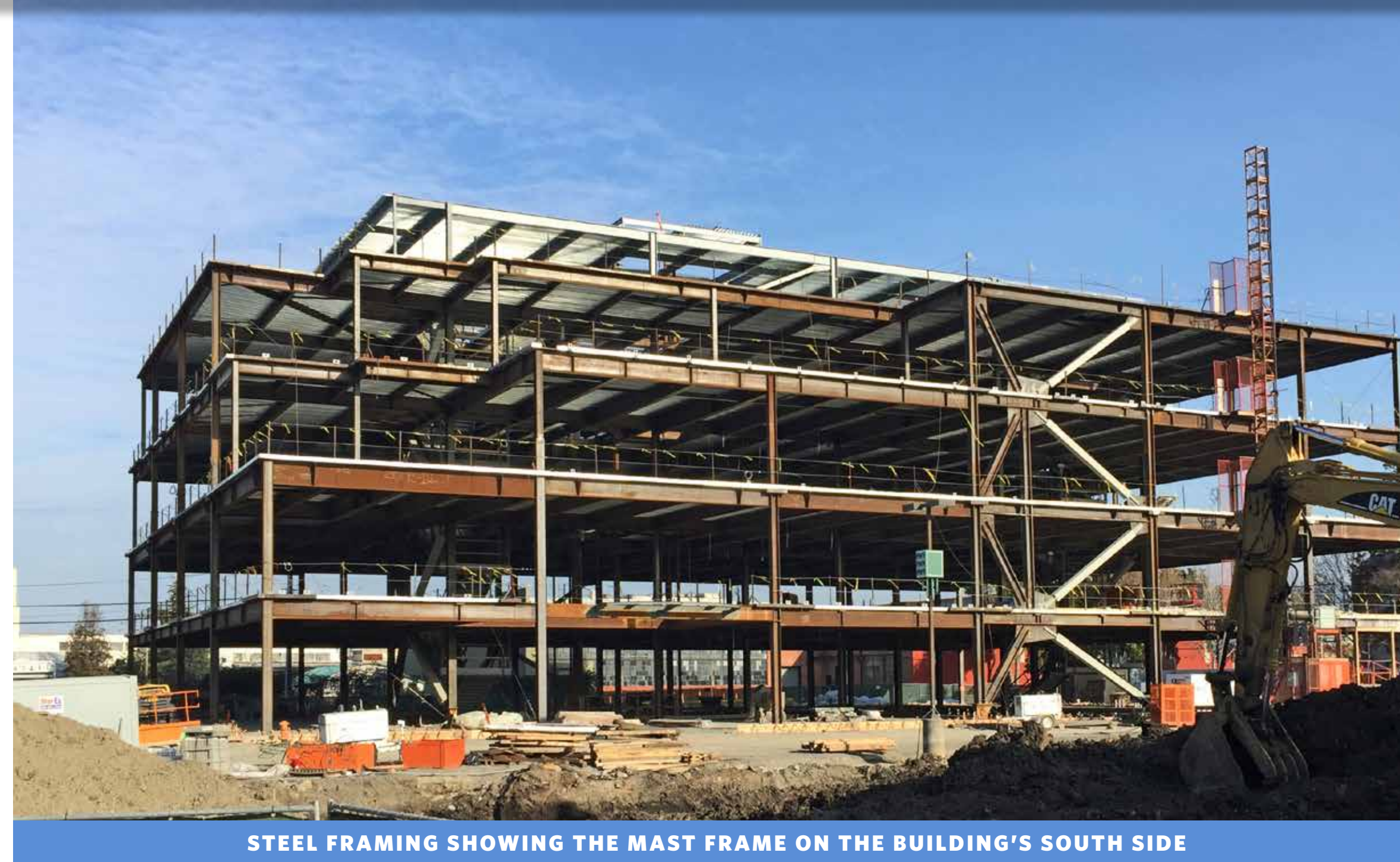
STEEL FRAMING SHOWING THE MAST FRAME ON THE BUILDING'S SOUTH SIDE
