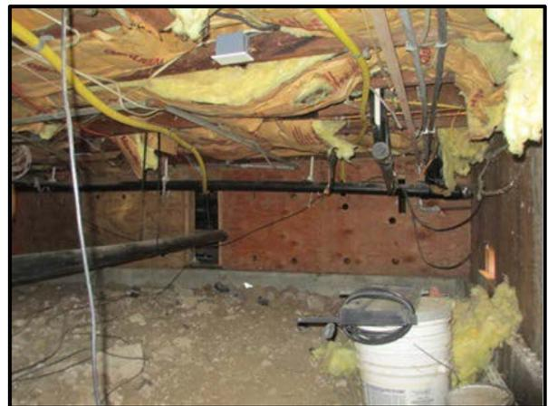
**Figure 2: Strengthened cripple wall in a crawl space, undamaged in the South Napa earthquake (Photo courtesy of ZFA Structural Engineers)**
