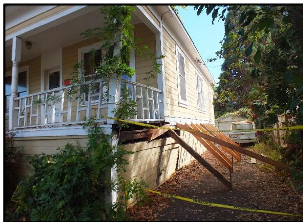
**Figure 1: Damaged cripple wall at the crawl-space level, braced on the outside to stabilize the dwelling and prevent collapse**
