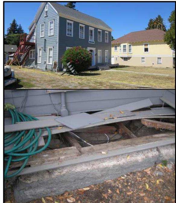
**Figure 3: Dwelling with damage to its cripple wall (top); failure of the cripple wall, resulting in the movement of the dwelling off its foundation (bottom) (Photo courtesy of ZFA Structural Engineers)**
