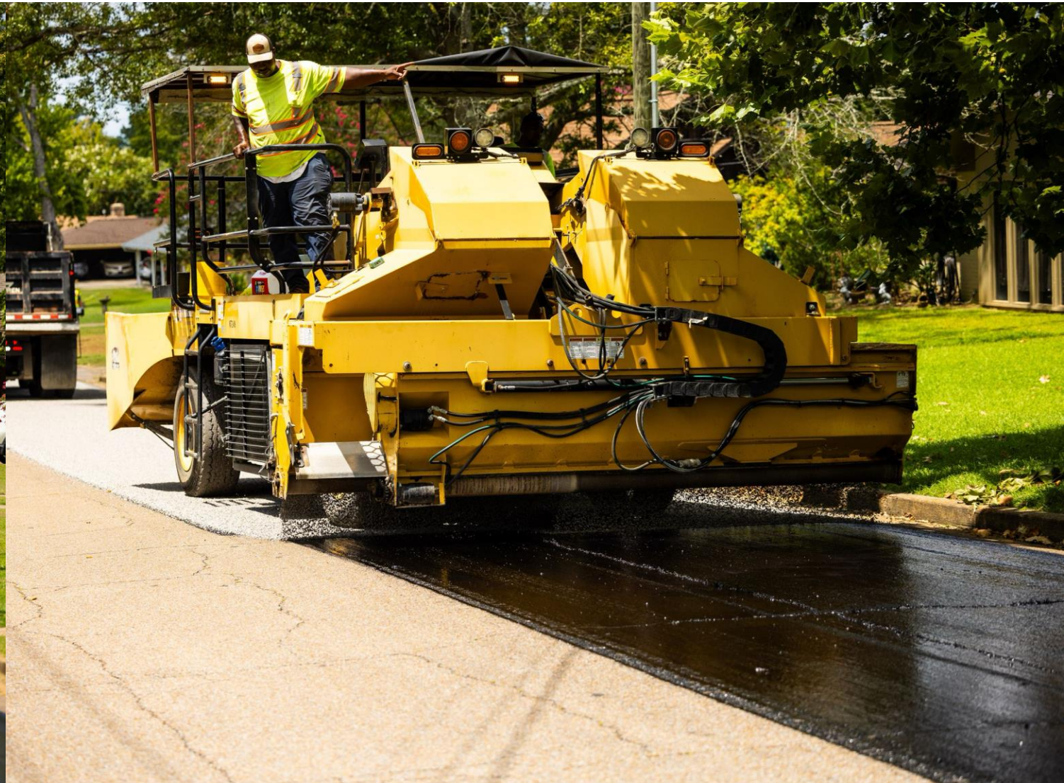
Rejuvenating Scrub Seal
