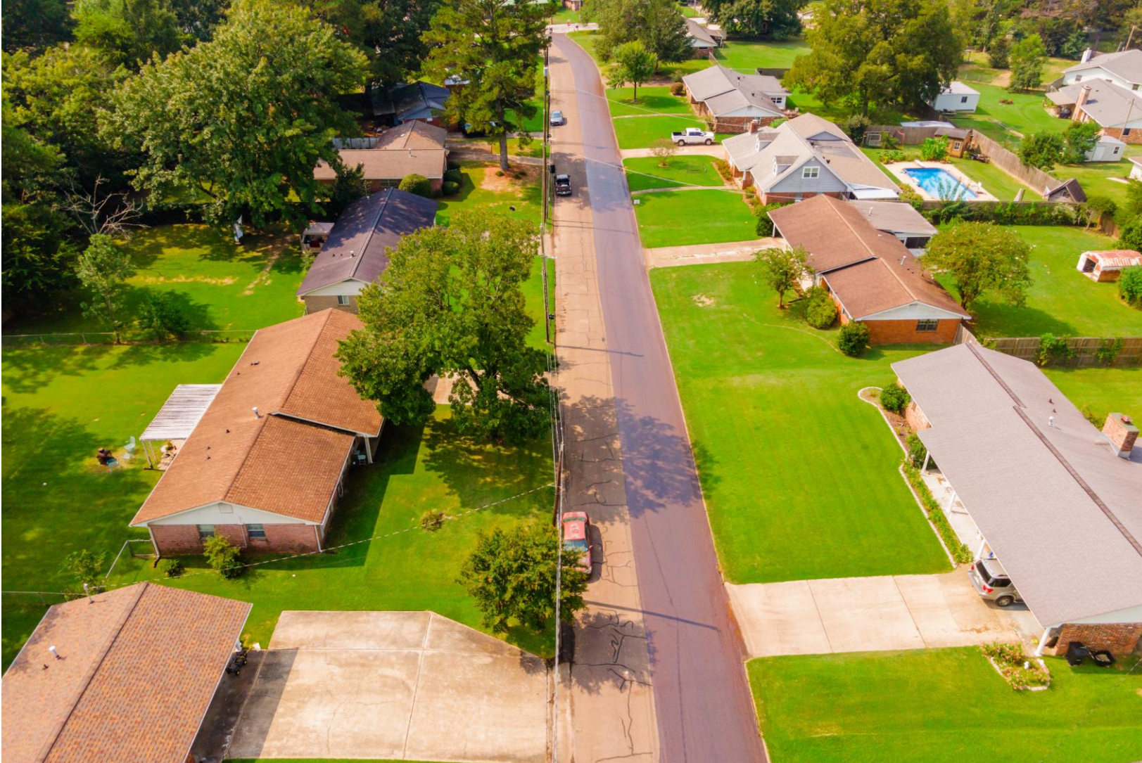
Crack Sealant + Highly Modified Micro Surfacing
