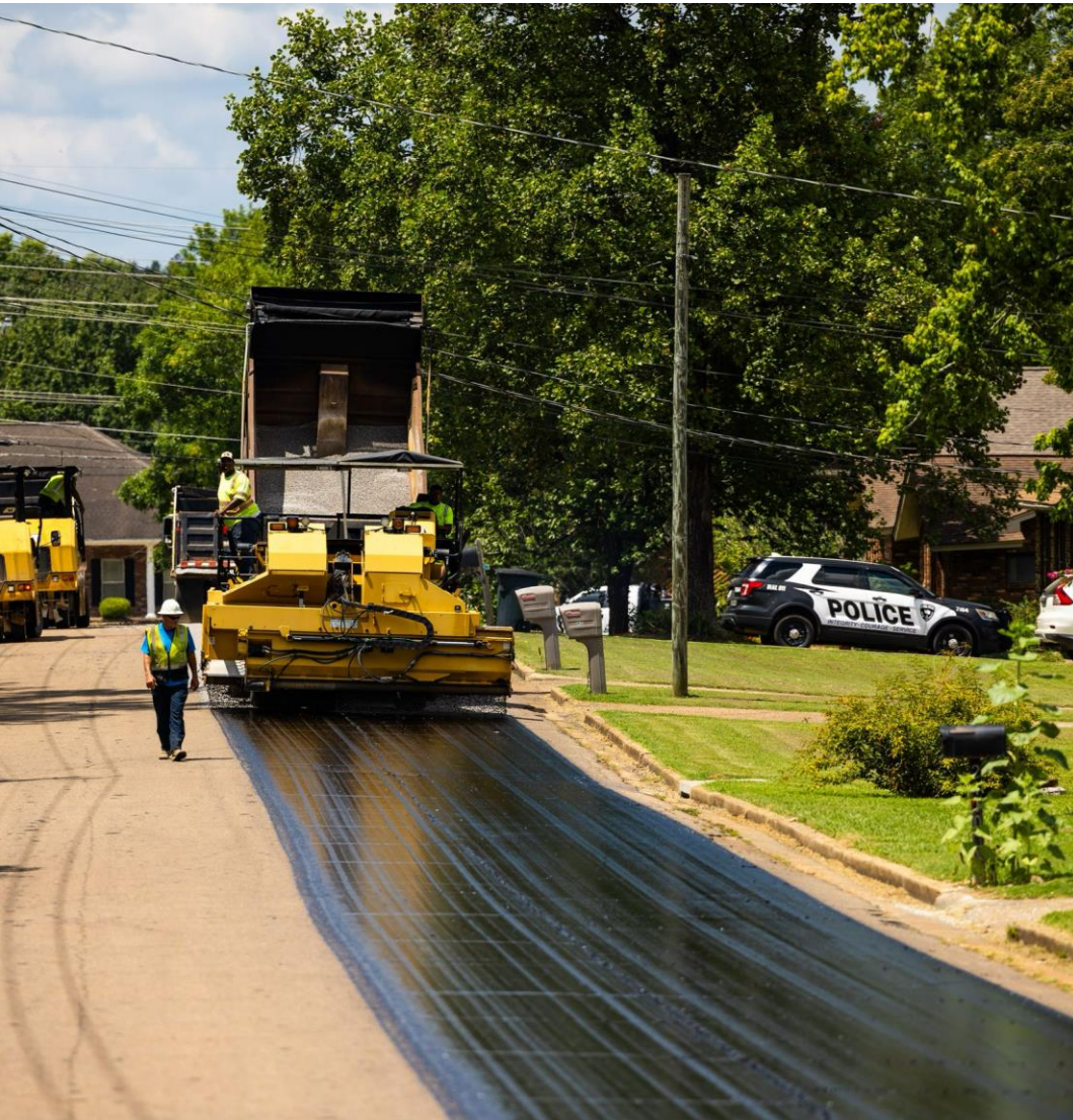
Rejuvenating Scrub Seal
