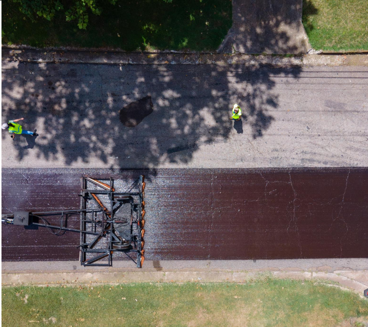
Rejuvenating Scrub Seal
