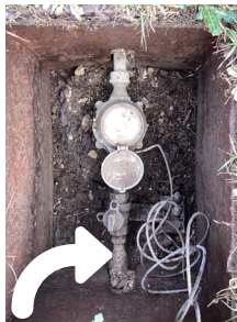
Replacing lead service lines like this one is part of the City of Waco Action Plan
