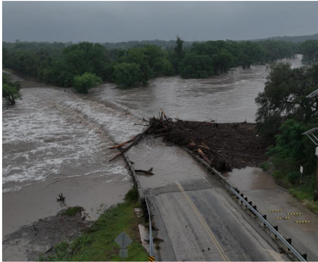
Guadalupe River floodwaters and debris overwhelm a rural Texas bridge.
