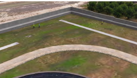
SURFACE MOUNTED FLOOD WALLS
