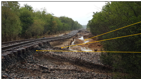
Image of Railroad Embankment after Failure
