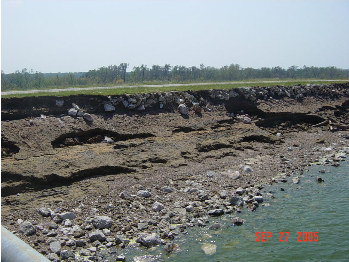
Figure 15: Lake Livingston Dam erosion and rip rap removal due to wave action. Source: NWS Houston/Galveston
