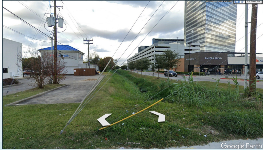
W157-00-00 at Westheimer (Looking South / Downstream)
