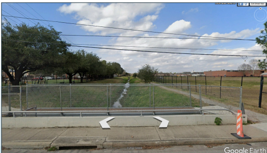
W157-00-00 at Briar Forest (Looking South / Downstream)
