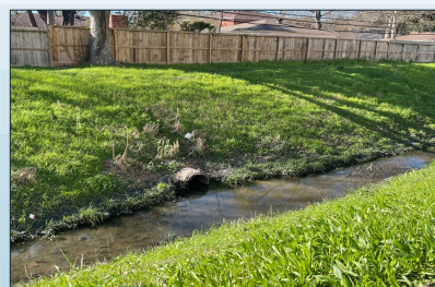
Low Outfall Pipes / Shallow Depths
