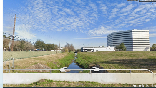
W157-00-00 At Del Monte (Looking South / Downstream)
