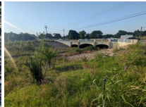
Stream Restoration at 28th Street
