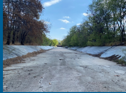
Downstream Concrete Channel
