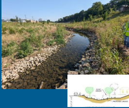
Downstream Stream Restoration
