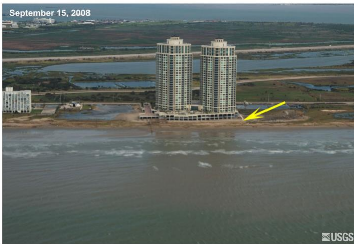
Palisades Palms Condominiums, Galveston Island. Before and after Hurricane Ike. Photo credit: coastal.er.usgs.gov
