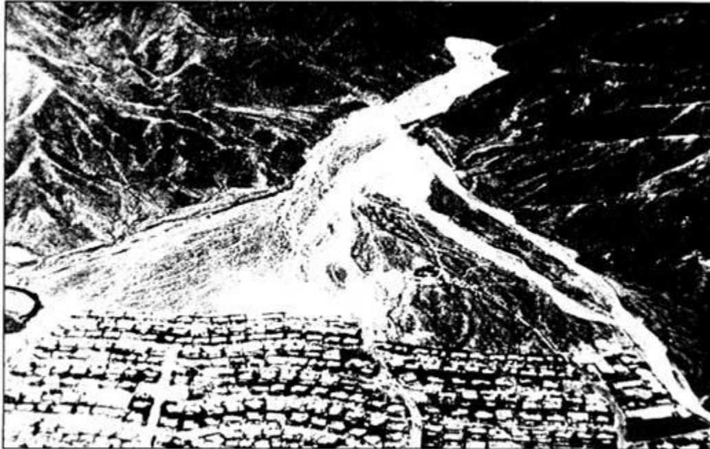
Figure 1-8. This alluvial fan flood caused over $7 million in damage and one death
