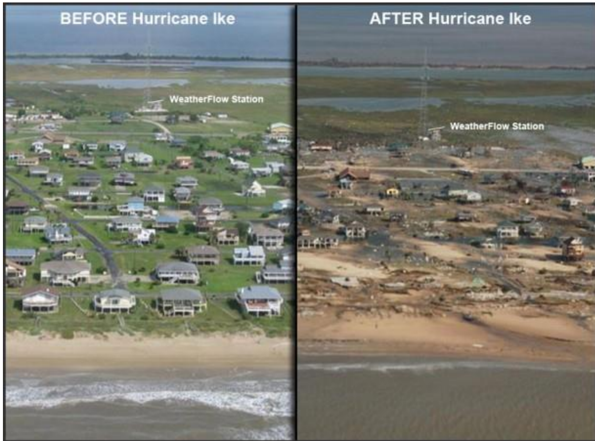
Bolivar Peninsula in 2008 before and after Hurricane Ike. Photo Credit: Weatherflow.com
