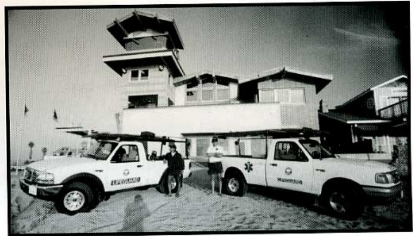
Imperial Beach Captain Robert Stabenow and seasonal LG-1 Oscar Alvarez in front of their new Safety Center.
