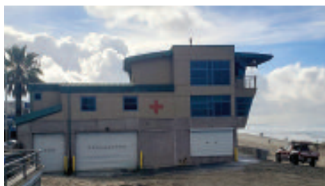
One of nine permanent oceanfront lifeguard stations with an enclosed observation deck on the third floor, offices and locker rooms on the second floor, garages and a medical aid room on the first floor. Photo: B. Chris Brewster
