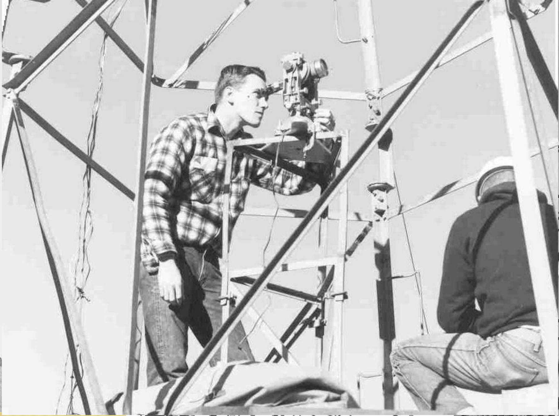
BILBY TOWER CONSTRUCTION
