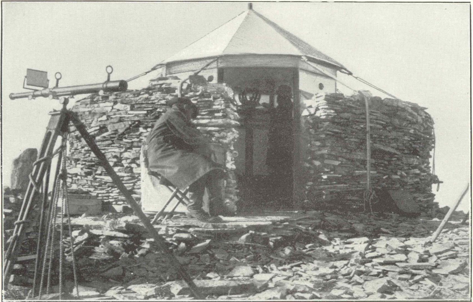
HIGH SUMMIT STATION, TUSHAR MOUNTAIN, UTAH, SHOWING RING WALL AND DOUBLE SHELTER TENT AGAINST STORMS AND RADIATION OF HEAT.
