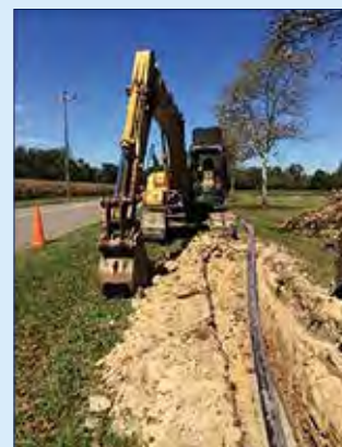
Figure 1: HRSD King William Treatment Plant conveys ~60,000 gallons of reclaimed water per day to Nestle Purina Petcare Company. Approximately two miles of six-inch pipe was installed during project construction in 2015-2016.
