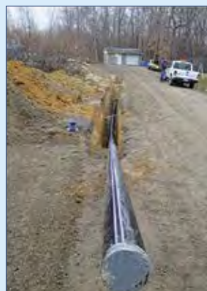
Figure 1: HRSD King William Treatment Plant conveys ~60,000 gallons of reclaimed water per day to Nestle Purina Petcare Company. Approximately two miles of six-inch pipe was installed during project construction in 2015-2016.
