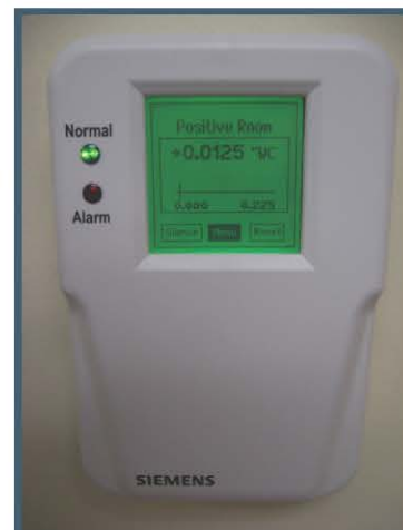
Alarmed manometers can warn staff of improper pressurization conditions.
